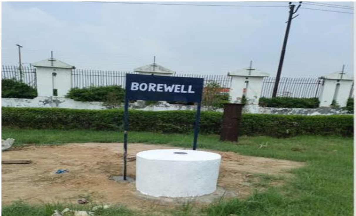
Sustainable water extraction from Borewell when required
